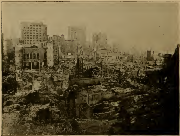
VIEW, LOOKING EAST, IN BALTIMORE AFTER THE GREAT FIRE.
